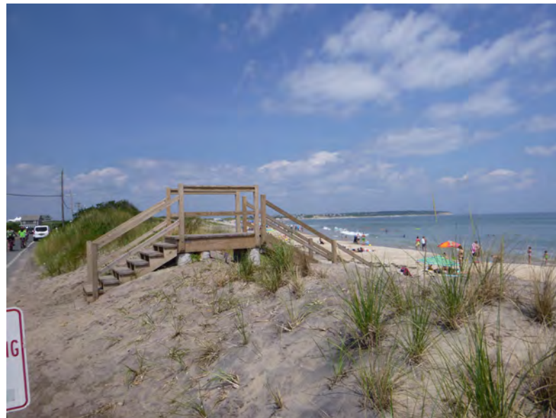
Removable stairs along Corn Neck Road providing safe access to the beach and protecting sensitive dunes from foot traffic
