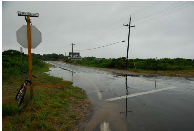
Ponding at intersection of Beach Road and Corn Neck Road
