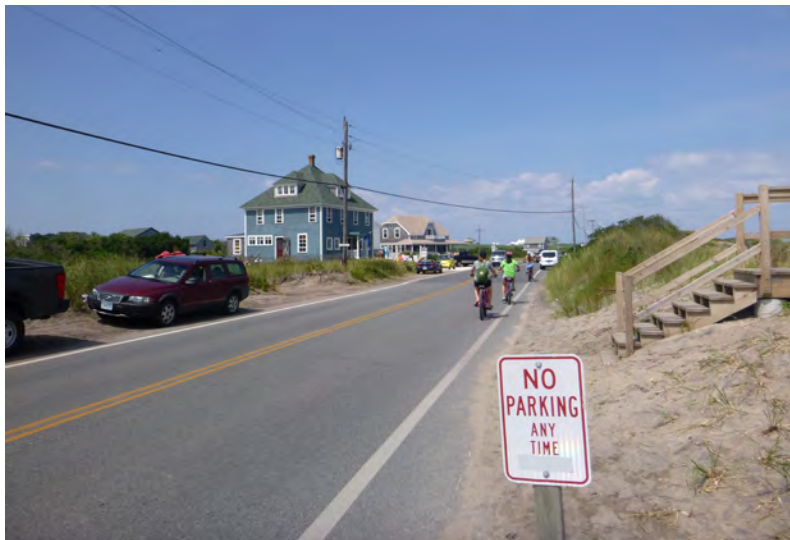
Reconstructed roadway and dunes along Corn Neck Road
